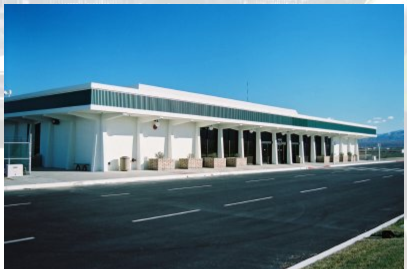
Palmdale Terminal Remodel Photo: Jay Berkowitz, LAWA.
